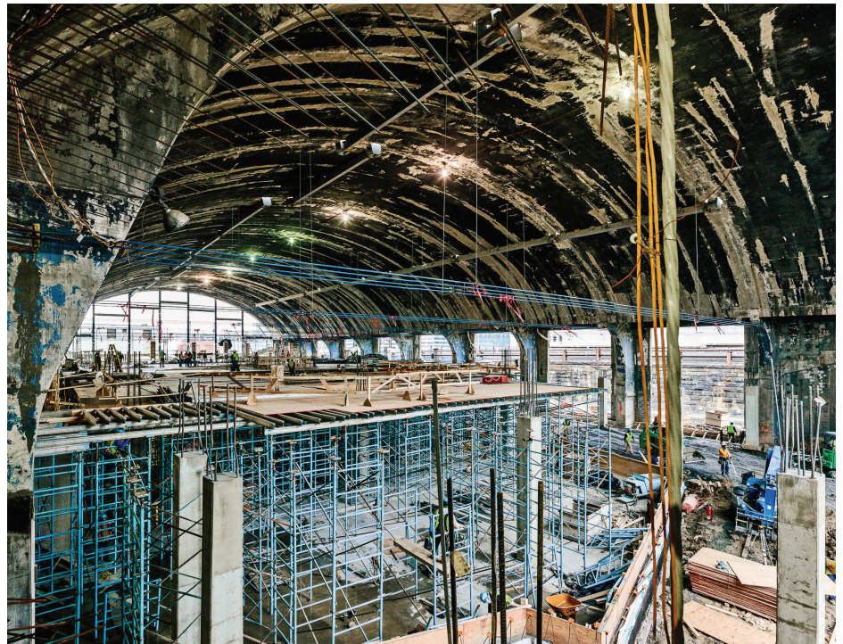
James G. Davis Construction Corp. (No. 83) is renovating Uline Arena, also known as the Washington Coliseum, in Washington, D.C. Built in 1941 and the site of the first Beatles concert in the U.S. in 1964, the facility will be the home to an REI flagship store as well as 174,000 sq ft of prime office space. ■
